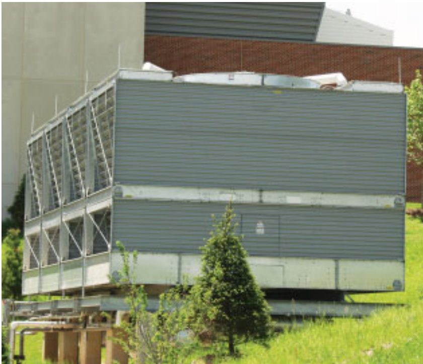
Multiple cooling tower cells for a central chilled-water plant.
